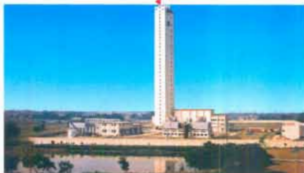
106 M Tower EHV Manufacturing Bay
