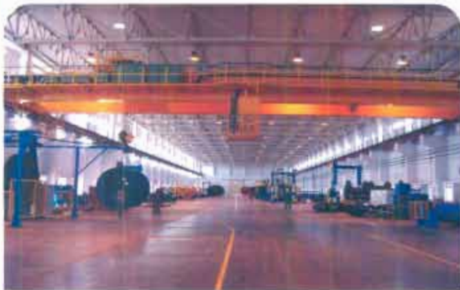
Internal View of VCV Plant →
